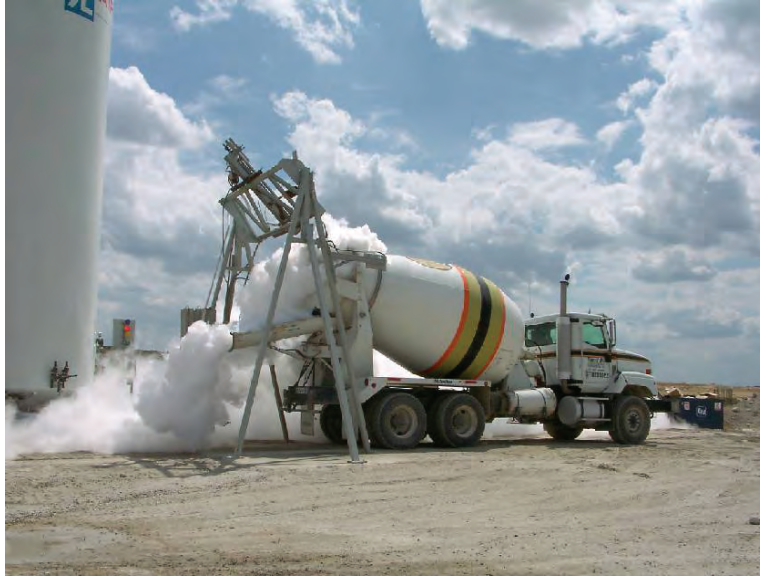
Figure 2.3 Cooling fresh concrete with liquid nitrogen
